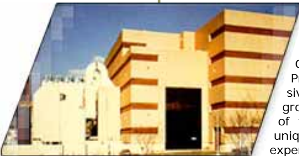
SCRRRA facility in Preston, CT
