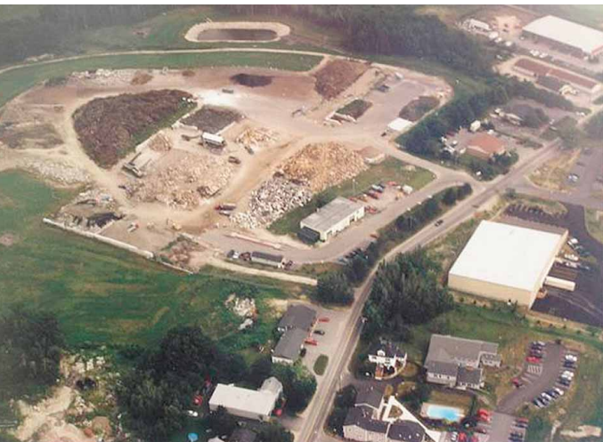
The Riverside Recycling Facility sits on top of a closed and capped bulky waste and construction and demolition debris landfill on the northwest side of Portland.
